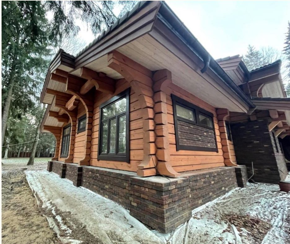
The flagship project: more than 700 square metres, built of 250 \times 350 mm pine beams
